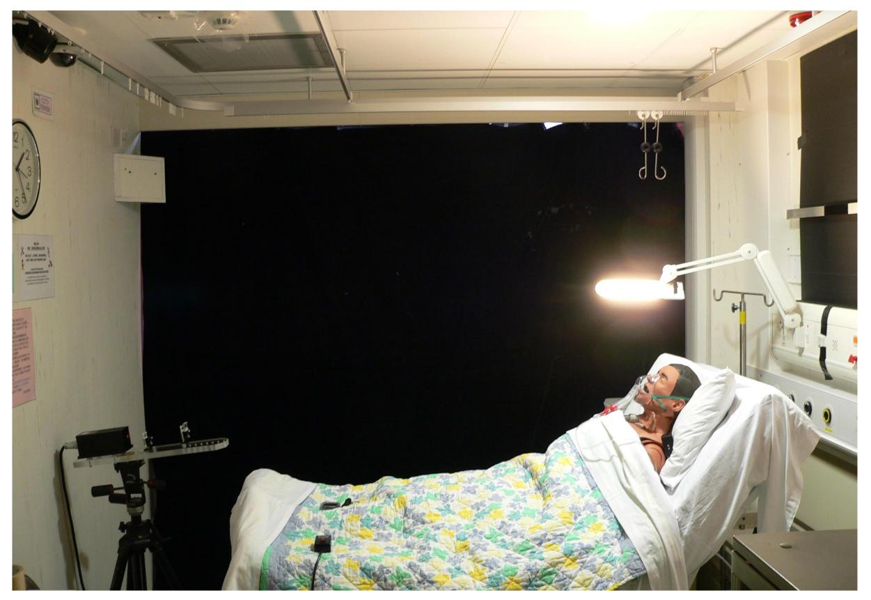
Figure: The more congested isolation room B at PWH, with air supply diffusers mounted on the ceiling at the foot of the patient bed and floor level exhausts underneath the head of the patient Dr. Benny CHOW bed.
