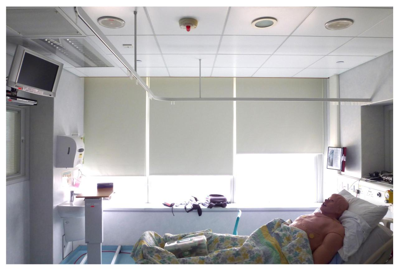
Figure: Spacious single bed patient room of isolation room A at PMH, with air supply diffusers mounted on the ceiling at the end of the patient bed and floor level exhaust underneath the head **Dr. Benny CHOW** of the patient bed.
